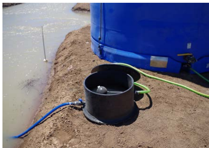
Example of a "header tank" for water running Urea 26.
